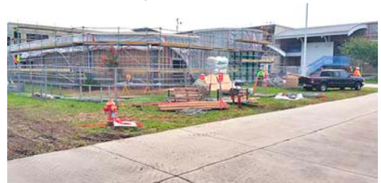
Modernizing and face lift inside and out for Azalea Middle School.
