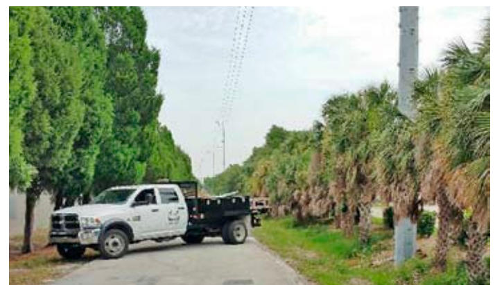
Strengthening Power Lines along Pinellas Trail.
