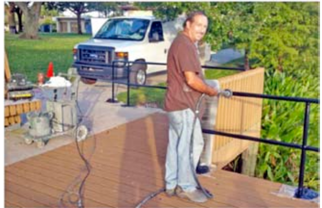
Railings on ALL Shelters NEW Paint by JOE, 35 years experience.
