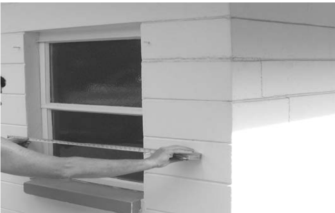
Here measures the width (above) and Height (below). Plywood comes in 4' by 8' sheets so plan accordingly.
