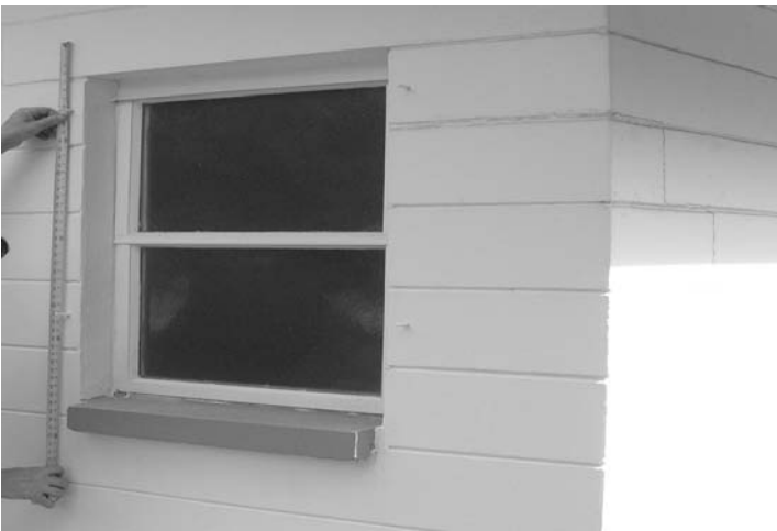
Here measures the width (above) and Height (below). Plywood comes in 4' by 8' sheets so plan accordingly.
