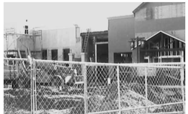
Construction in progress on Bonefish Grill and Lee Roy Selmon's Restaurants.
