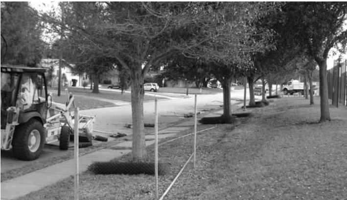
Removal of old fence.
