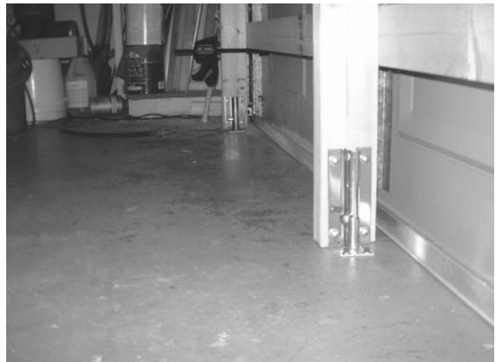
To keep things simple and fast I used heavy duty gate catches on the ends of the vertical 2x4's. You will need a hammer drill to make the hole in the garage floor for the gate catch pin.
