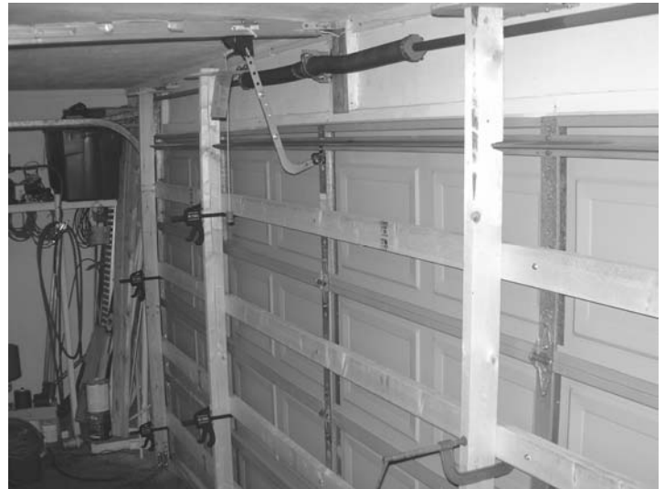
I decided that I needed four vertical 2x4's. When installed I used clamps to hold them to the horizontal 2x4's.
