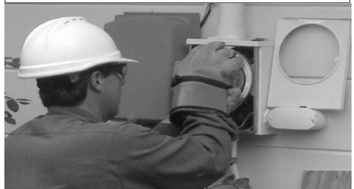
Progress Energy employee at work replacing the new radio frequency digital meters in our neighborhood.
