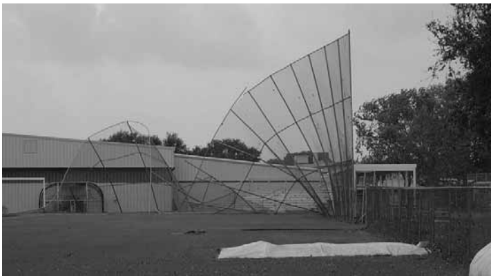
One of the practice backstops at Raymond A. Naimoli Baseball Complex suffered severe wind damage.
