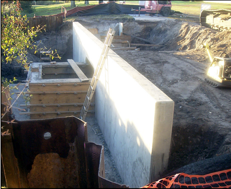
Storm Drain Project Reaches Destination
