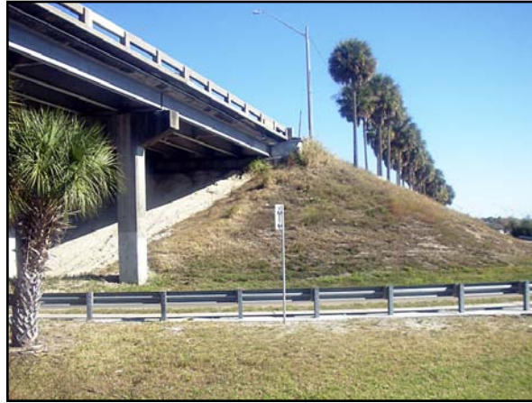
TYRONE OVERPASS all cleaned up for the Holidays
