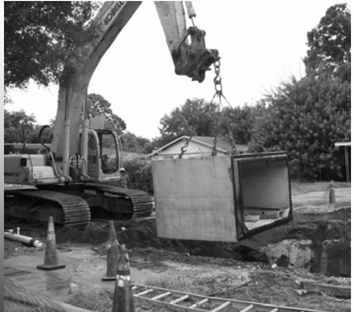
In Goes the Drain!
