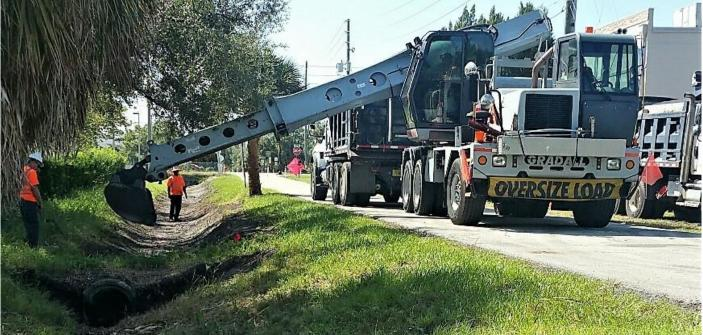
**Placed Grass Sod to bottom of Ditch!**
