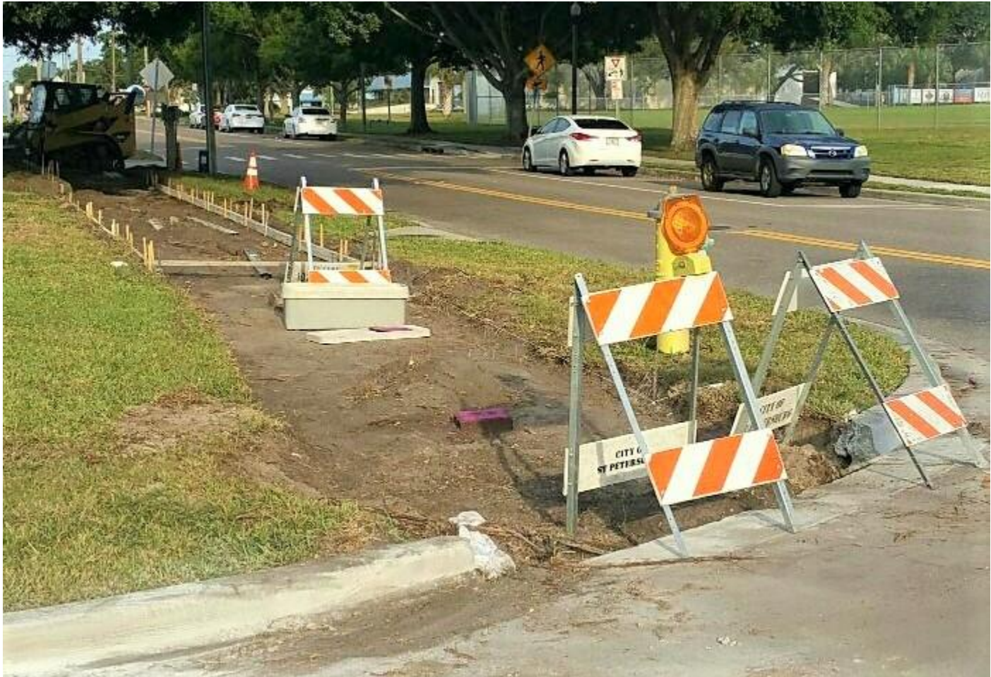
Sidewalk with ADA ramp at PARC
