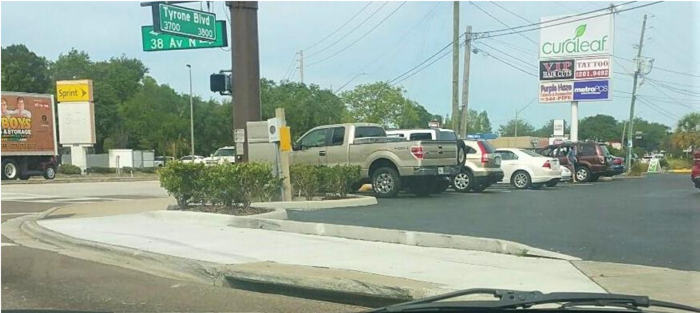
Infill Sidewalk 38 th Av at Tyrone. Was dirt and weeds.
